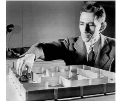
Electromechanical mouse that “solves” mazes! →
